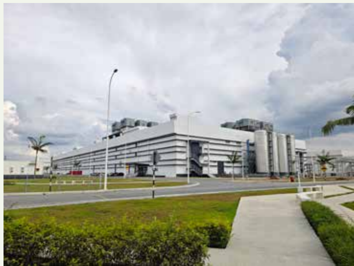
秦淮数据中心实景 Groundbreaking of Data Centre (Johor Bahru) Projects
